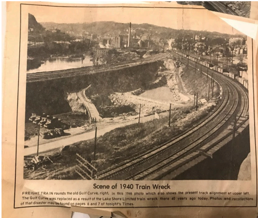
Old and new gulf curve during construction. Photo courtesy of the Little Falls Historical Society.
